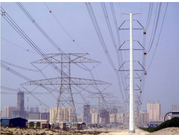
Figure 6: 400 kV compact line (right) parallel to a 400 kV conventional line (left), DEWA, UAE
